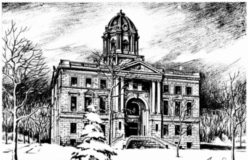
Old West Virginia State Capitol Annex Building -- Now Kanawha County Public Library
