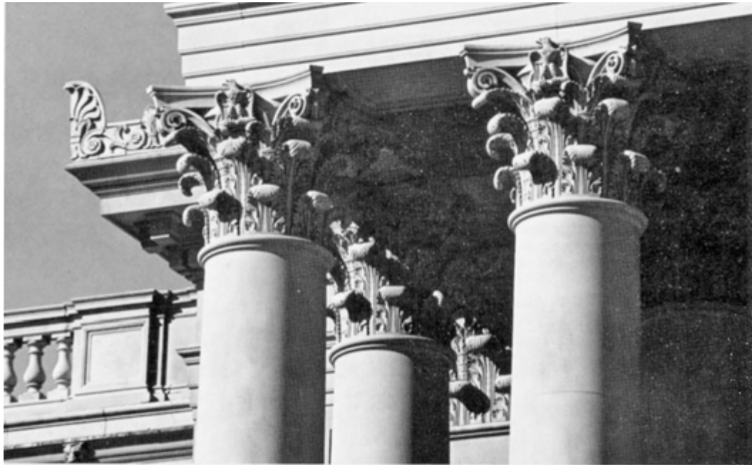
Above: Corinthian column caps, south portico.
