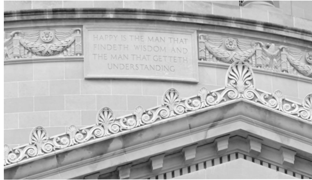
Ornamental terra cotta trimming the south pediment, and distinctive stone carvings below columns at base of dome.
