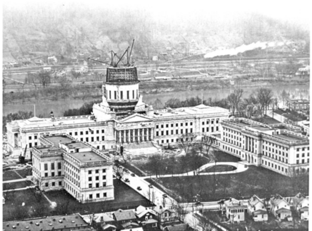
Opposite left: Main Building excavation site, July 1930. Center, both pages: Superstructure and preliminary stonework, November 1930. Top right: Southwestern corner of Main Building, January 1931. Above: View of complex from north, March 1931.
