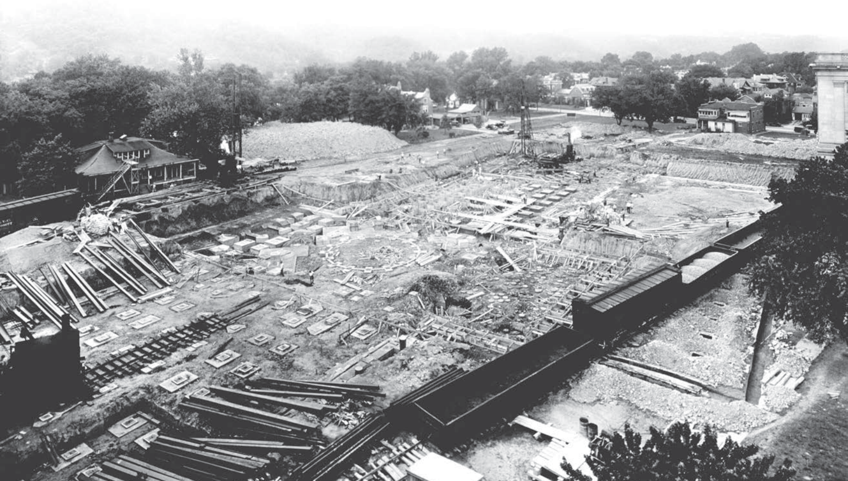
Main building excavation site, July 1930.
