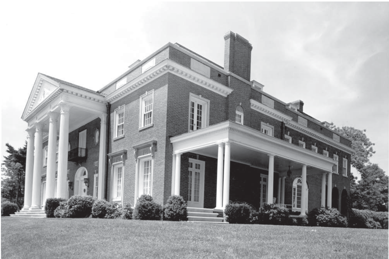
Above: The present Executive Mansion. Opposite page: West Wing superstructure, May 1924.
