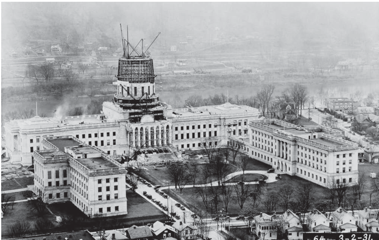
Left: Southwestern corner of Main Building, January 1931. Above: View of Complex from north, March 1931.
