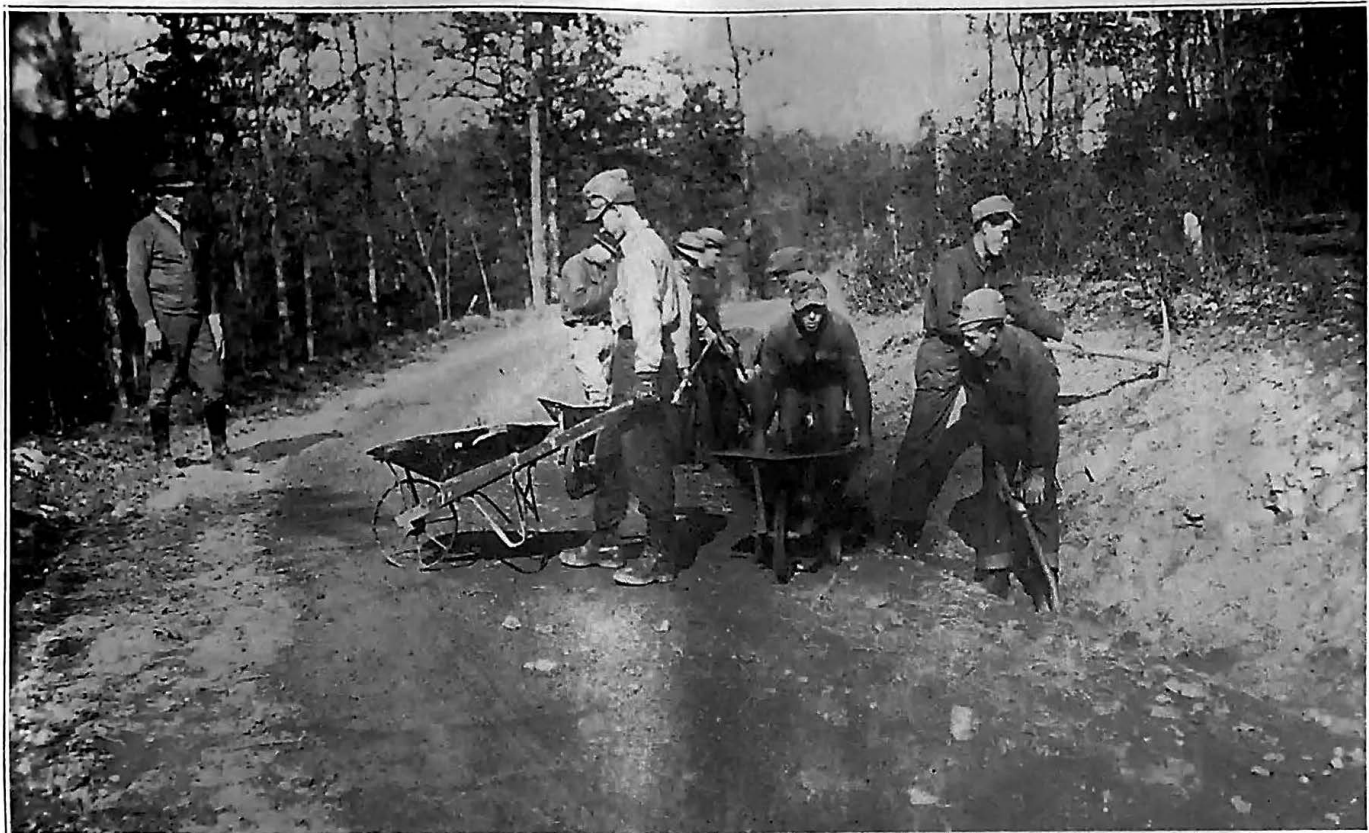
CCC Workers Building Mountain Road In West Virginia.
