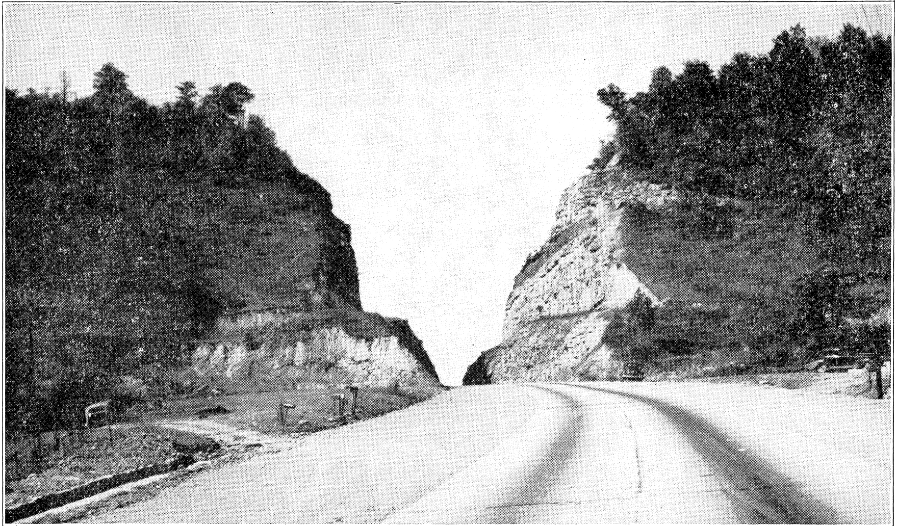
Deep highway cut, U. S. Route 52 atop Premier Mountain near Welch
