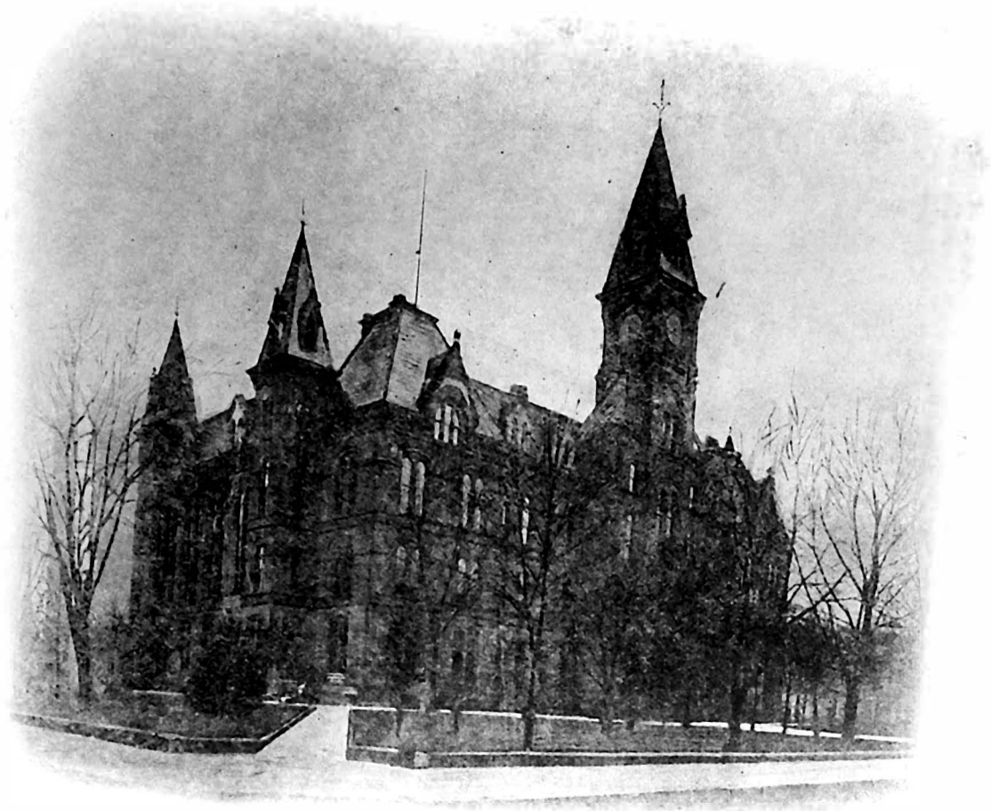
THE STATE CAPITOL AT CHARLESTON.
