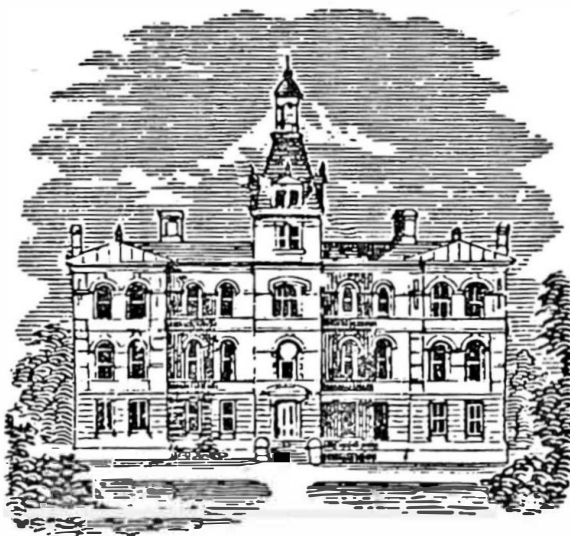
SECOND STATE CAPITOL BUILDING OF WEST VIRGINIA (First in Charleston)
