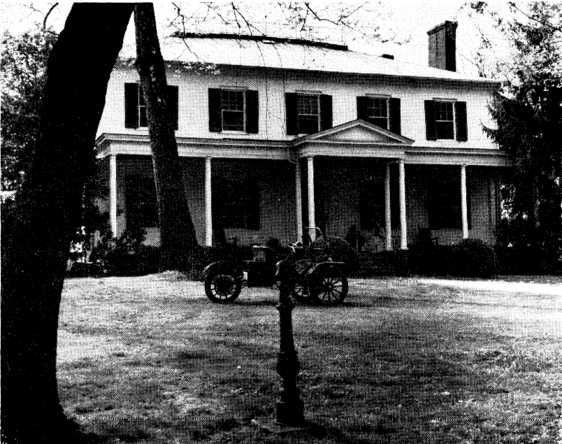
Boydville, in Martinsburg, Berkeley County, originally built in 1812. Most of the hardware and furnishings came from England, including the wallpaper. The home was renovated and enlarged in 1900.
