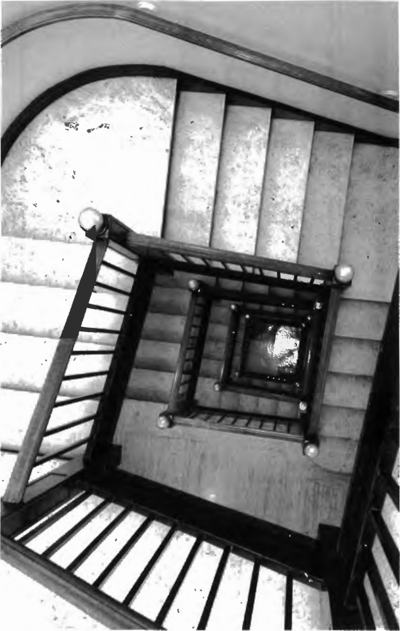
LOOKING DOWN THE STAIRCASE ON THE NORTHWEST SIDE OF THE CAPITOL MAIN UNIT.
