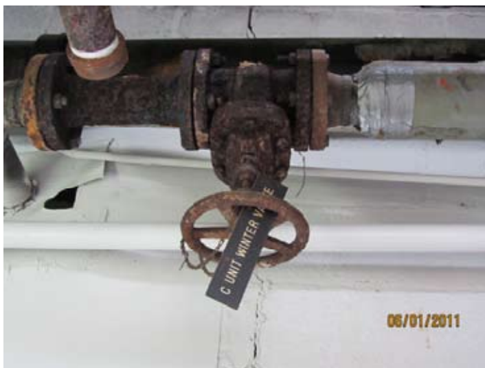
Existing Steam valves are failing.
