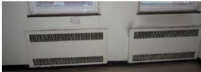
Existing Typical P-TAC Type Units
