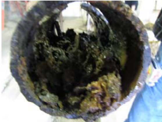
Existing Restricted Flow Sanitary Line
