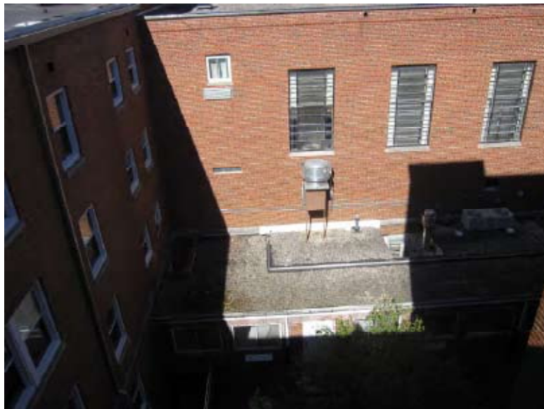
Kitchen Hood Exhaust system venting into operable window.
