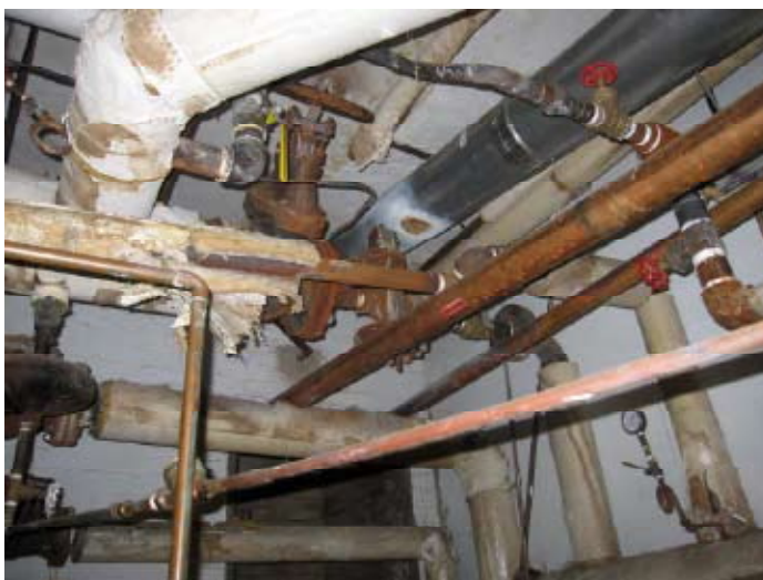
Existing Steam Distribution Piping
