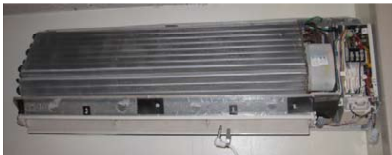
Terminal Type Air-Conditioner (Non-Functional)
