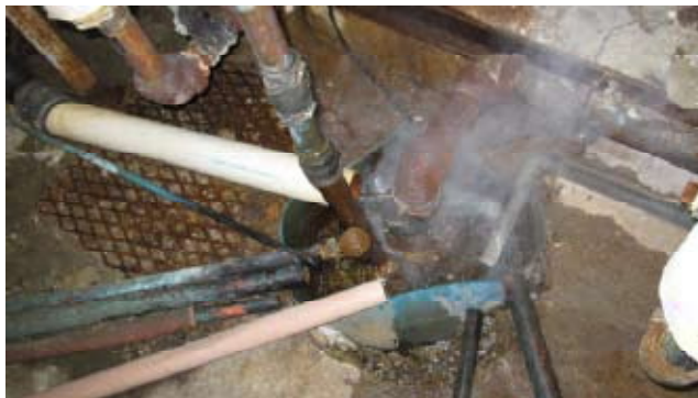
Existing Overflow and drain piping to sump pump
