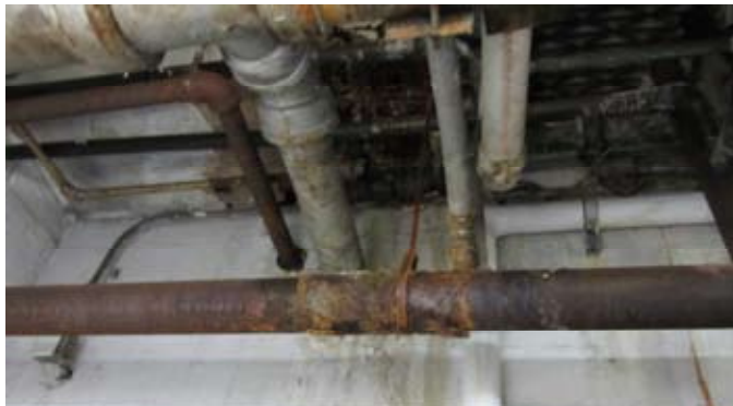
Deteriorated Sprinkler Piping
