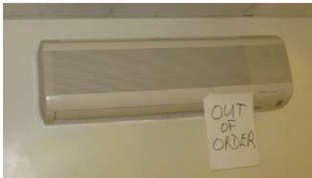
Existing Typical Split System (Non-Functional)
