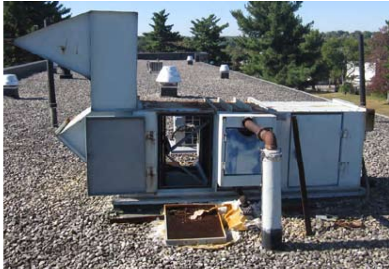
Existing RTU (Non-Functional).
