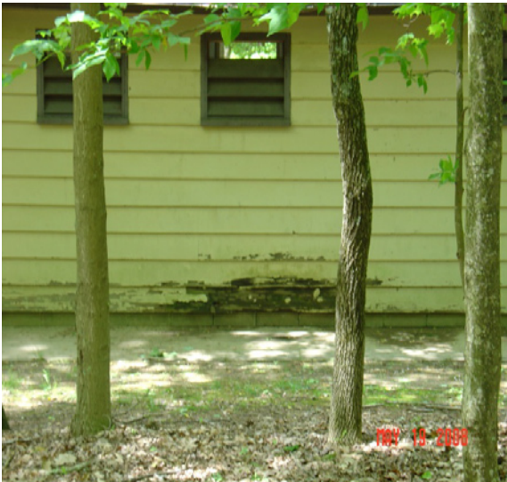
North Bend State Park Bathroom
