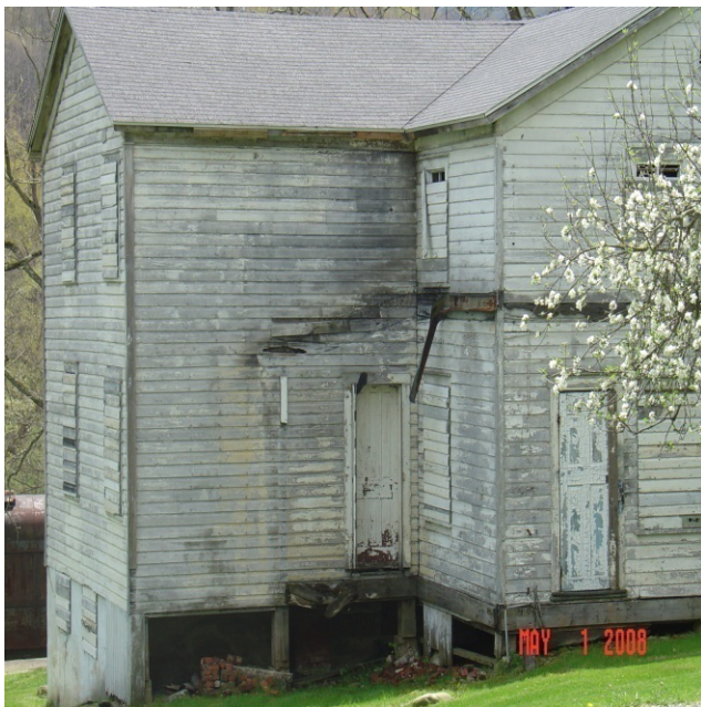
A Viable Cass Logging Home in Need of Repair
