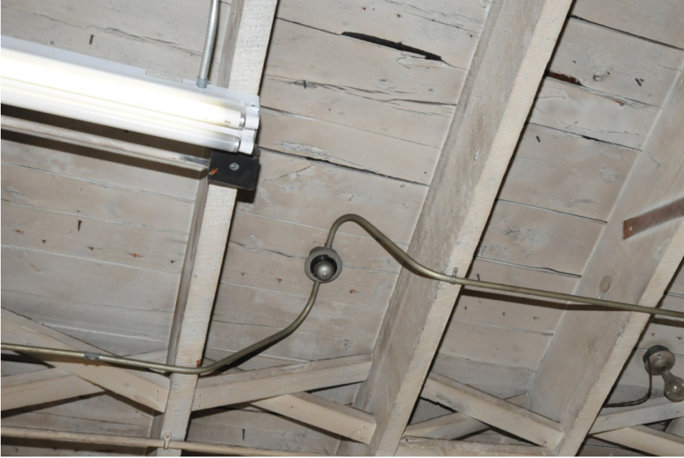
Electrical wiring attached to wood roof
