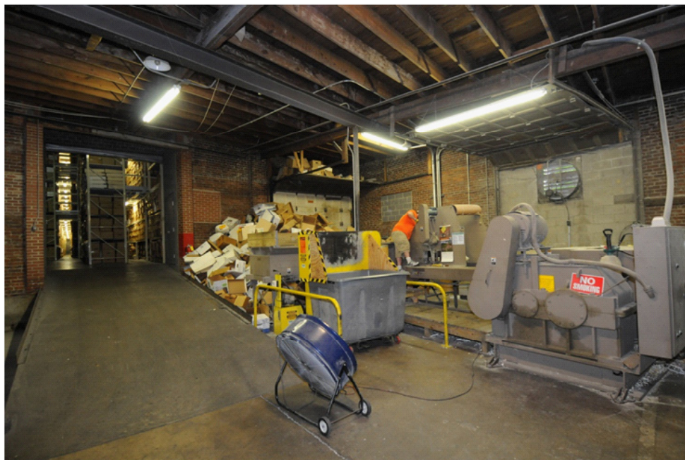
NOVA Facility Shredding Area
