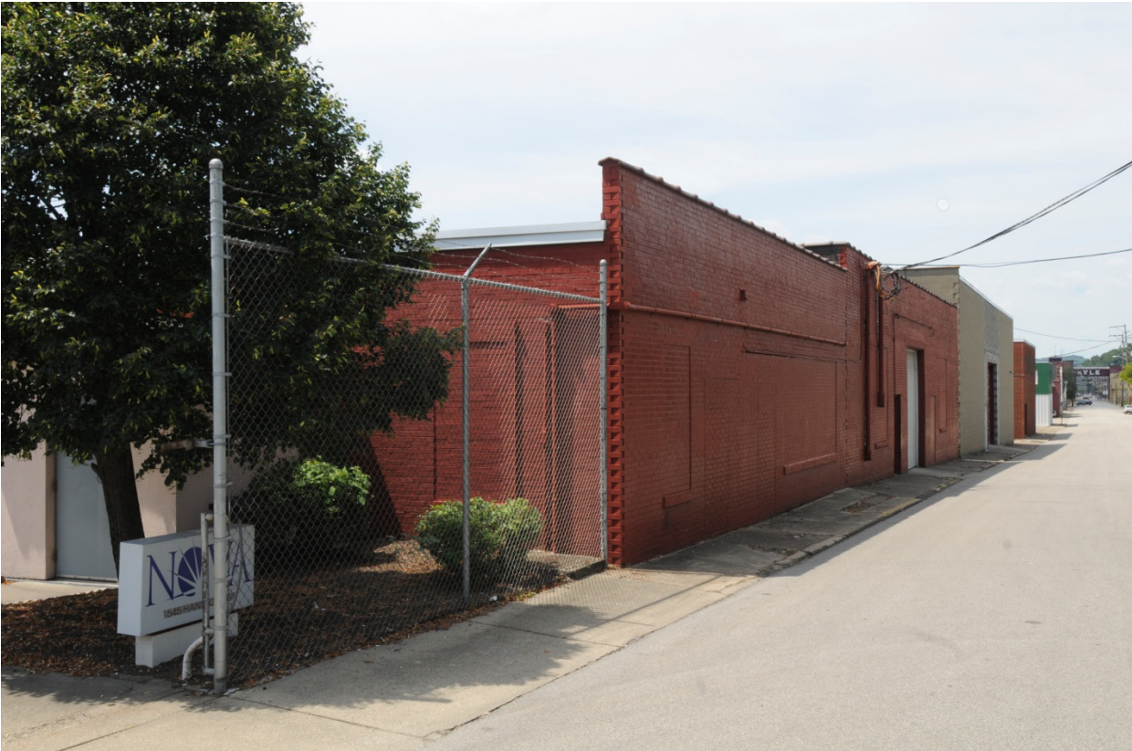
Exterior of NOVA Records, LLC, Charleston Storage Facility
