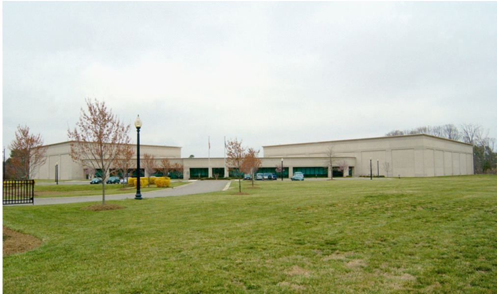
Exterior of Virginia Records Center
