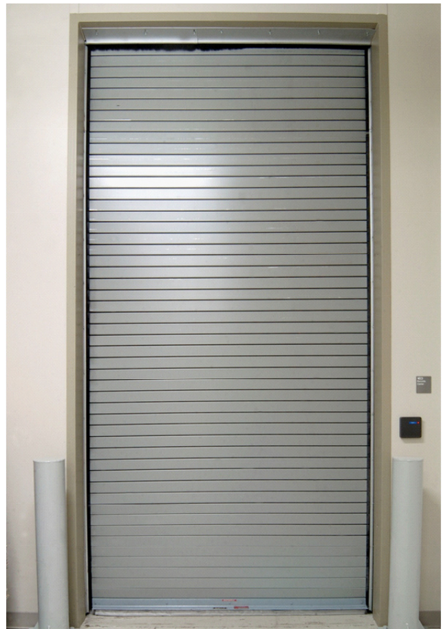
Loading Dock Door at Virginia Records Center
