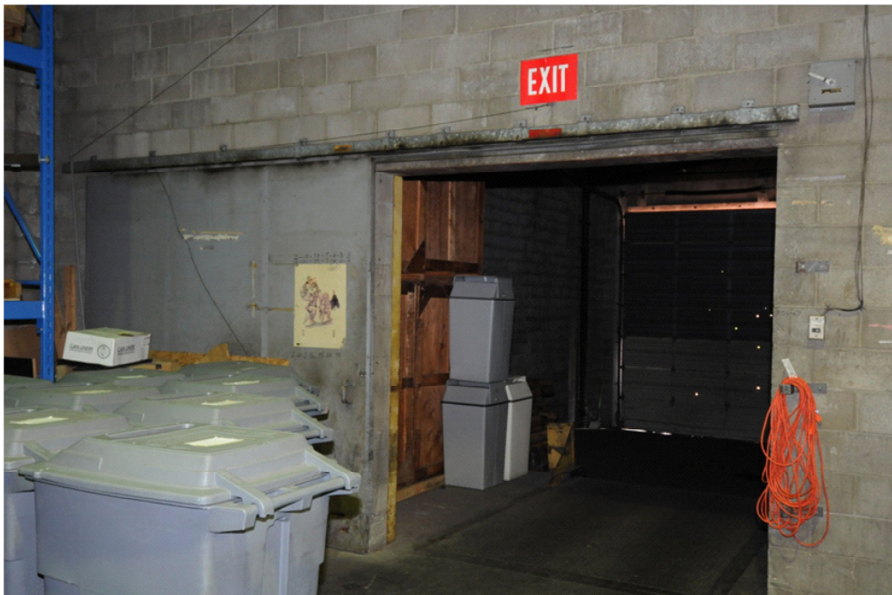
Loading Dock Door With Multiple Holes
