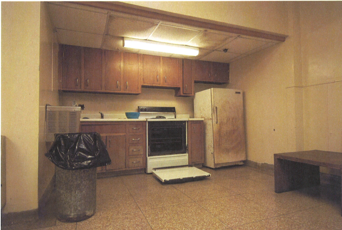
Rust on appliances and damage to ceiling tiles in Coed Hall.
