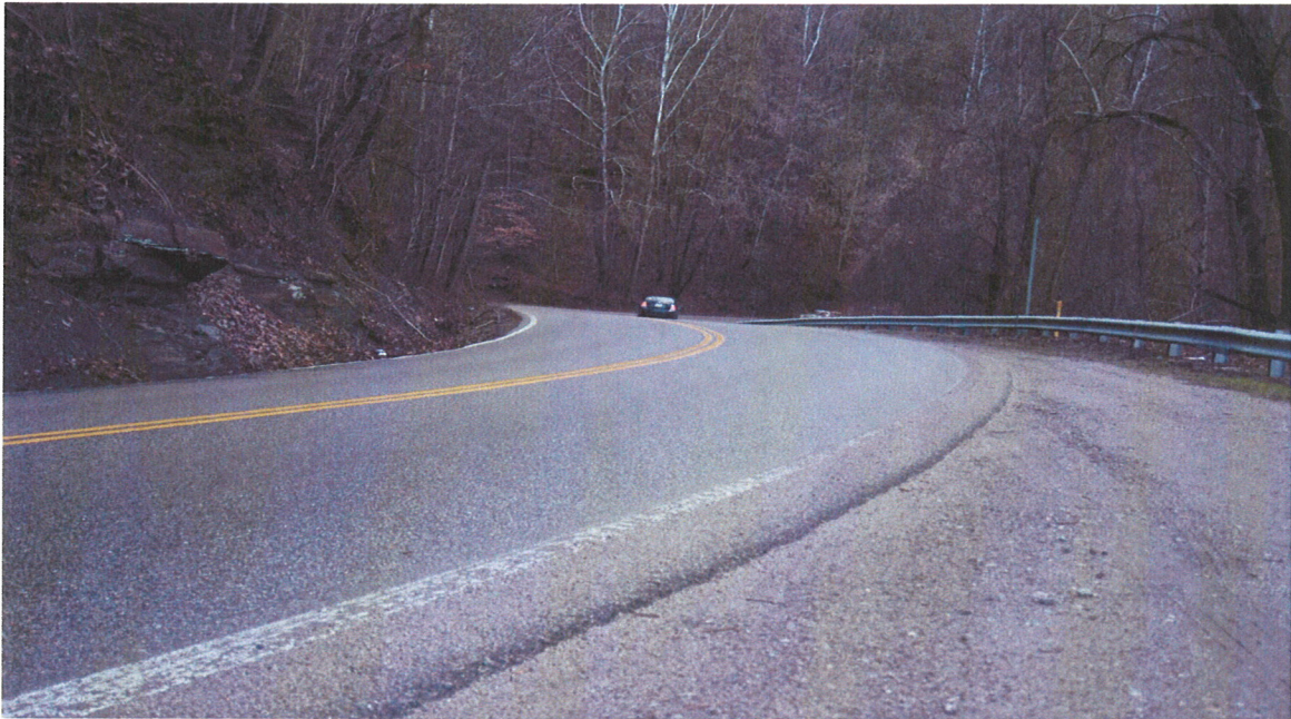
Route 61 (Fayette Pike) is a steep, narrow, winding roadway. This scene is taken going west away from Montgomery.
