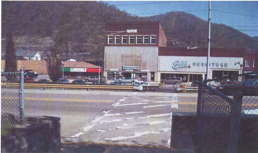
WVU Tech students must cross Rt. 61 and the railroad tracks to reach the business section of Montgomery from Old Main.
