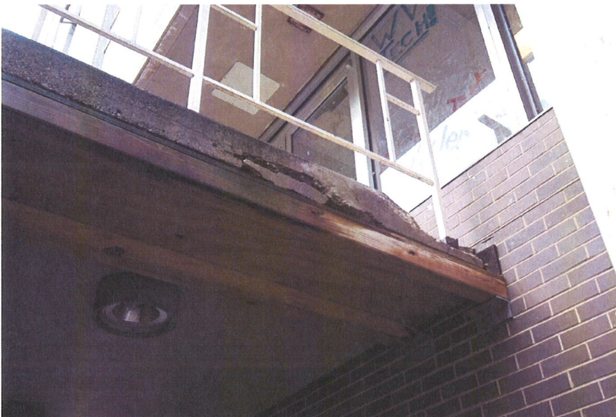
Exterior damage at Hirise.
