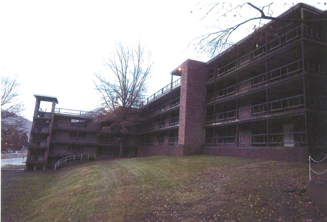
Coed Hall is no longer used due to structural damage and water incursion.
