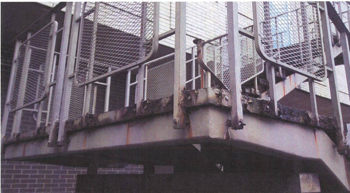
Damaged stairwell on the exterior of Hirise residence hall.
