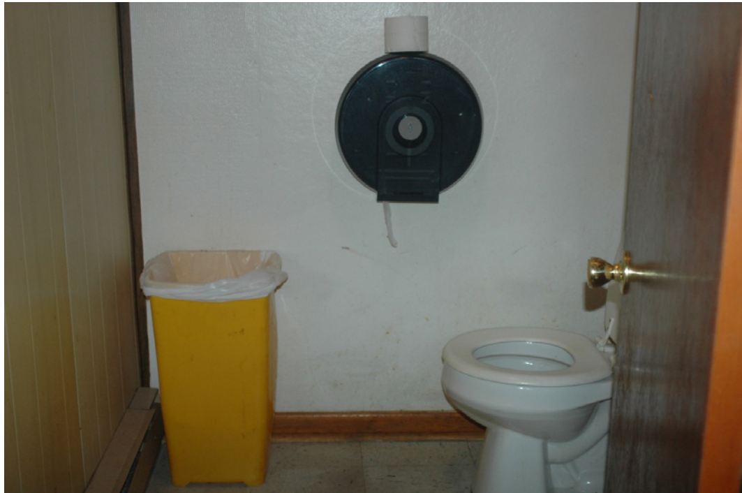
Figure 5: The small size of the Moorefield office’s restroom fails to meet most of the ADA’s measurement requirements, and is not accessible to veterans with a physical disability.
