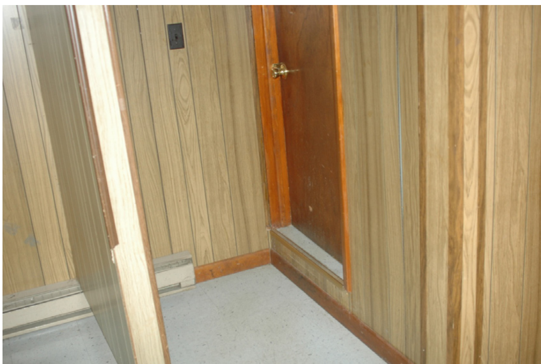
Figure 4: The Moorefield office does not provide an accessible restroom facility for veterans. As seen here, a veteran in a wheelchair could not even enter the restroom, due to the step-up at the door.
