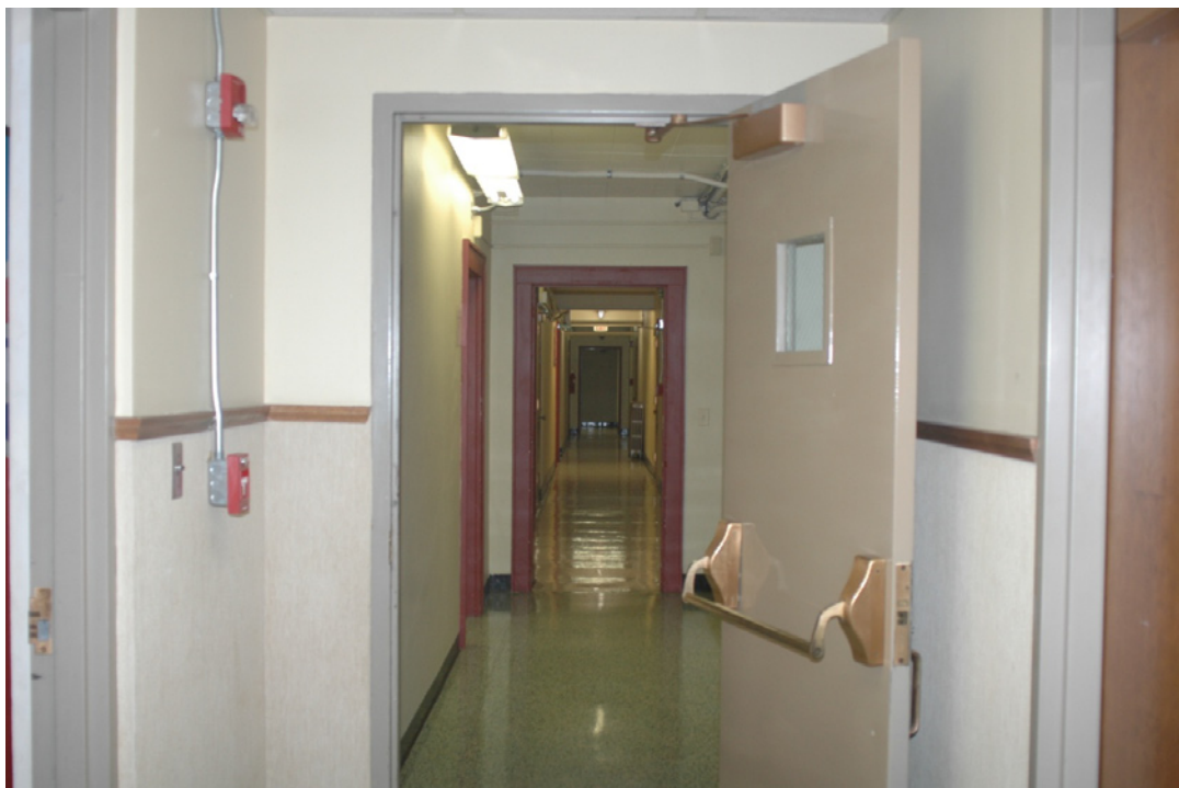
Figure 3: The narrow doorways and corridors at the Lewisburg office can make wheelchair navigation difficult for veterans. Some doorways (as seen above) fail to provide the ADA-required amount of clear space.
