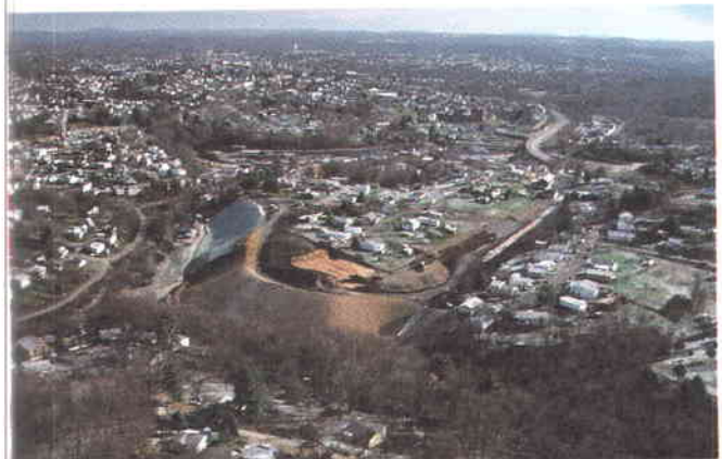
The Mabscott Project - Reclamation work in an urban setting.
