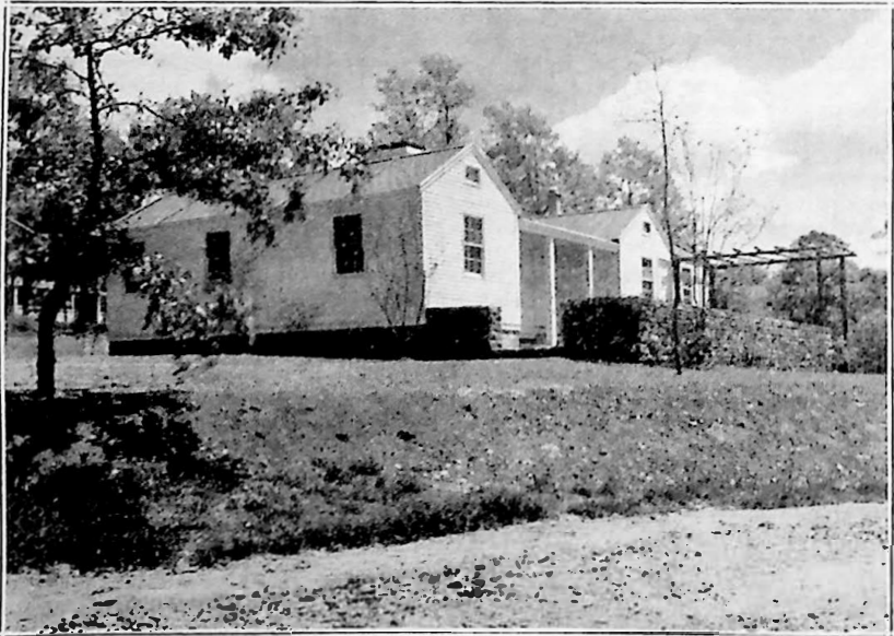
Type of home being erected at federal homestead project at Reedsville
