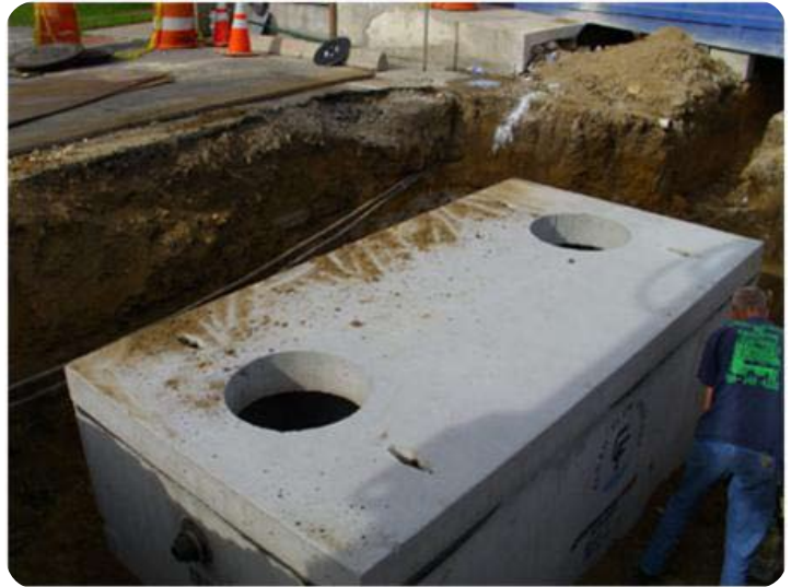
2000 Gallon Grease Trap Interceptor Project: Due to the increase in population at BCC, a larger grease trap interceptor system had to be installed.
