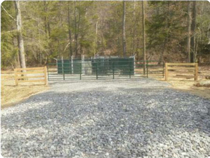
New Water Source Project: ACC continually had issues with pumping enough water to supply the facility. A new well was located and they are now able to pump enough water to supply the facility.
