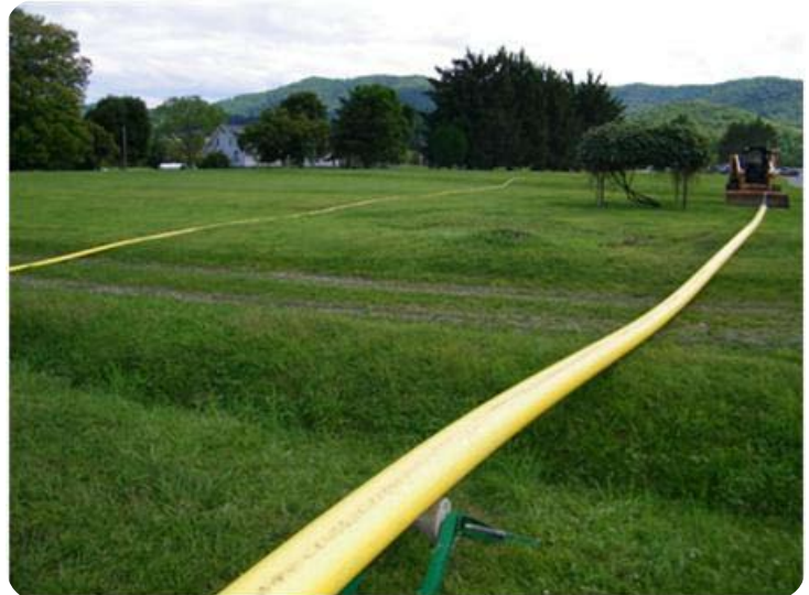
In-House Natural Gas Line Project: HCC had a natural gas line installed to the property line of the facility. For the facility to connect to the new service, the installation of the new line had to be completed to each area of the facility to connect to natural gas service. Once the line was installed, HCC converted all of their units operating off of fuel oil and LP gas to natural gas for energy savings.
