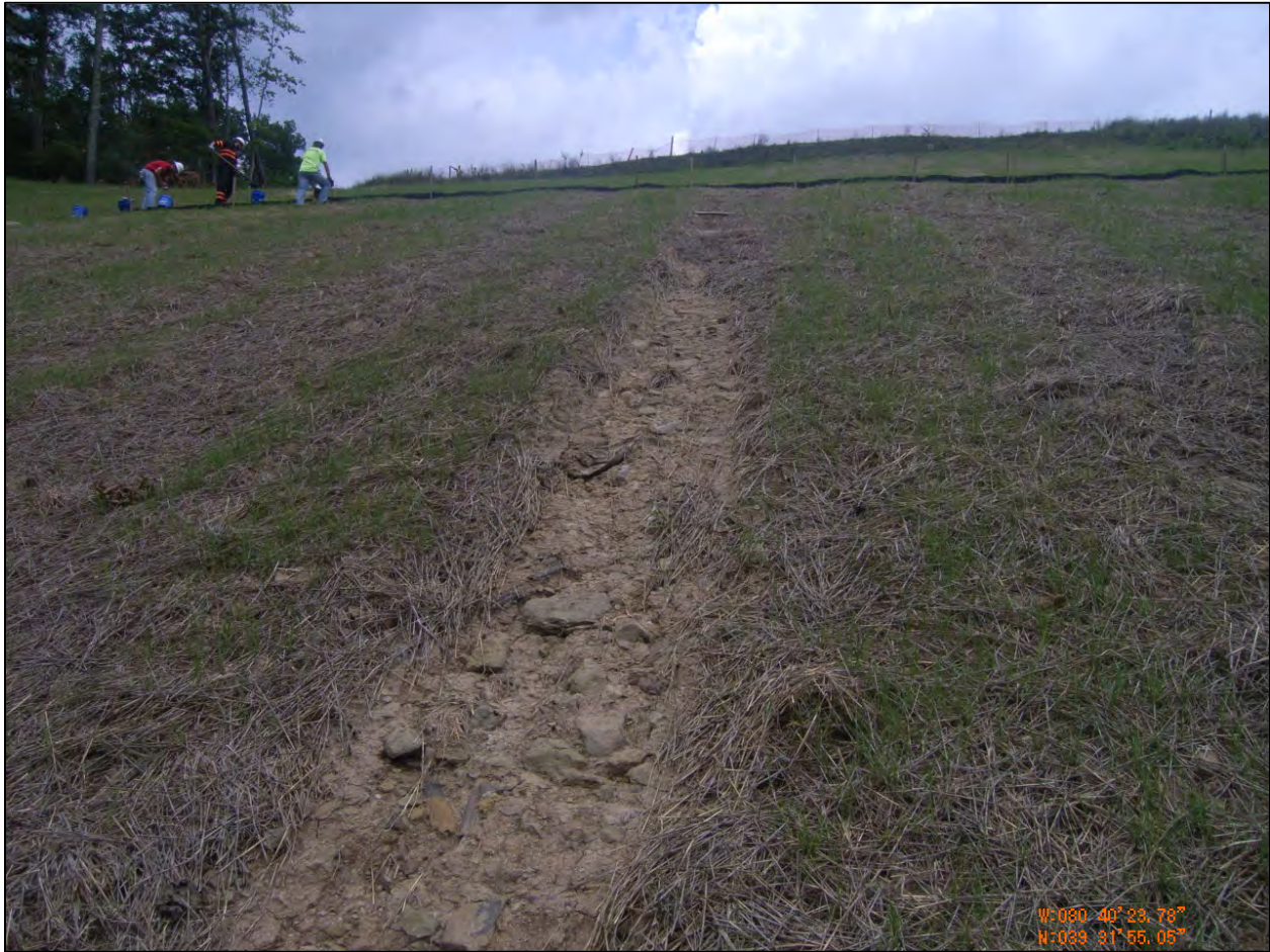
Figure 12: Surface Erosion at Mills-Wetzel
