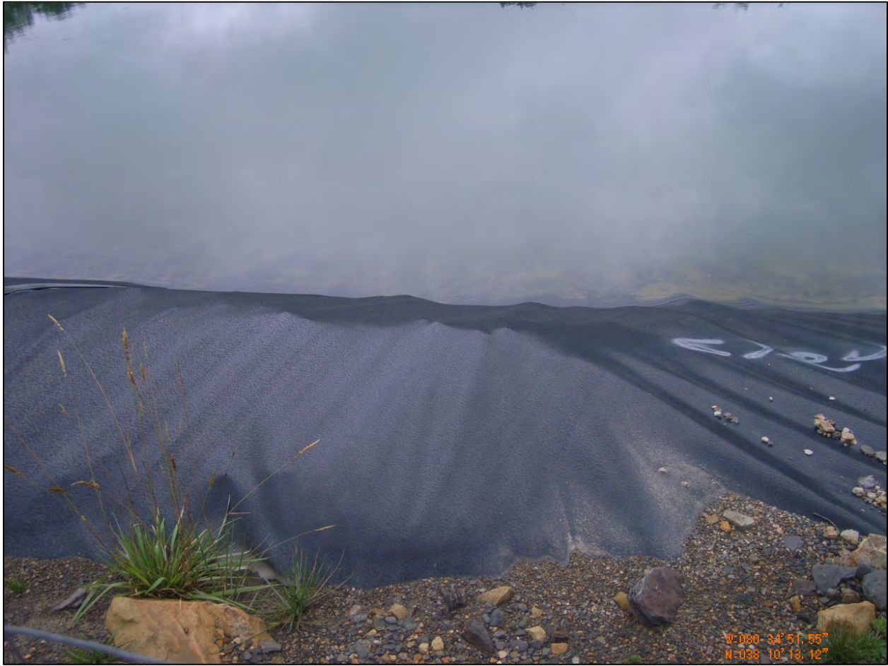
Figure 16: Liner Bulges at MWV
