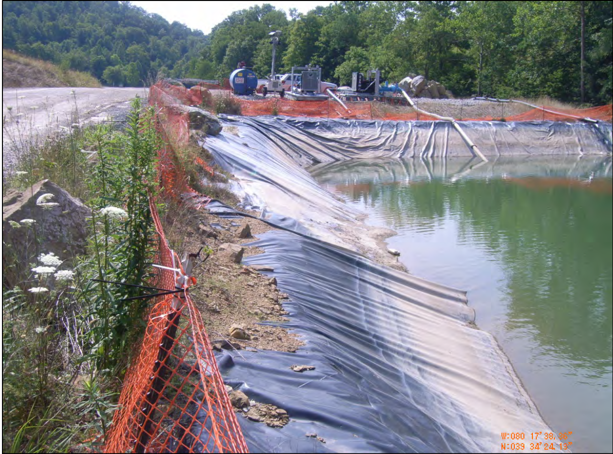
Figure 8: Rock and Debris on Liner
