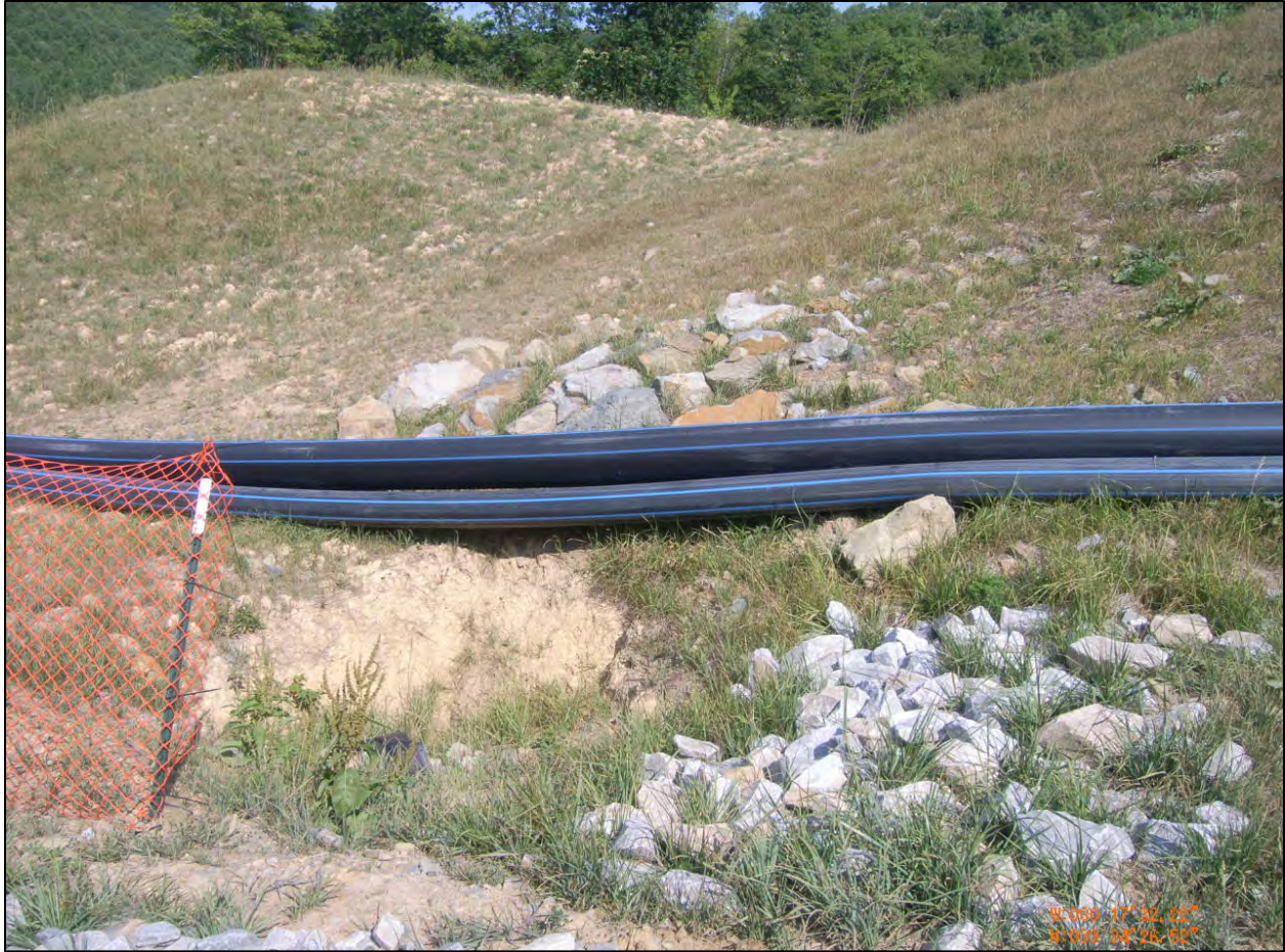
Figure 10: Unsupported Pipe
