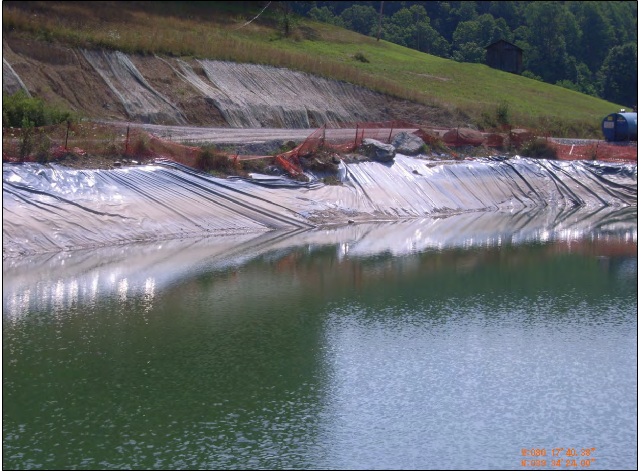
Figure 6: Slope Movement into Impoundment
