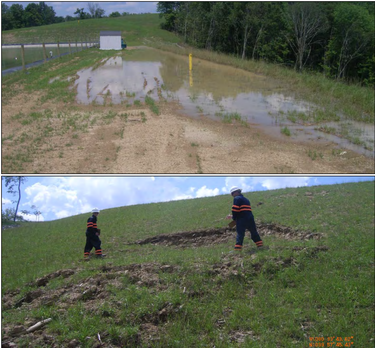
Figure 13: Slope Movement at SHL 4
