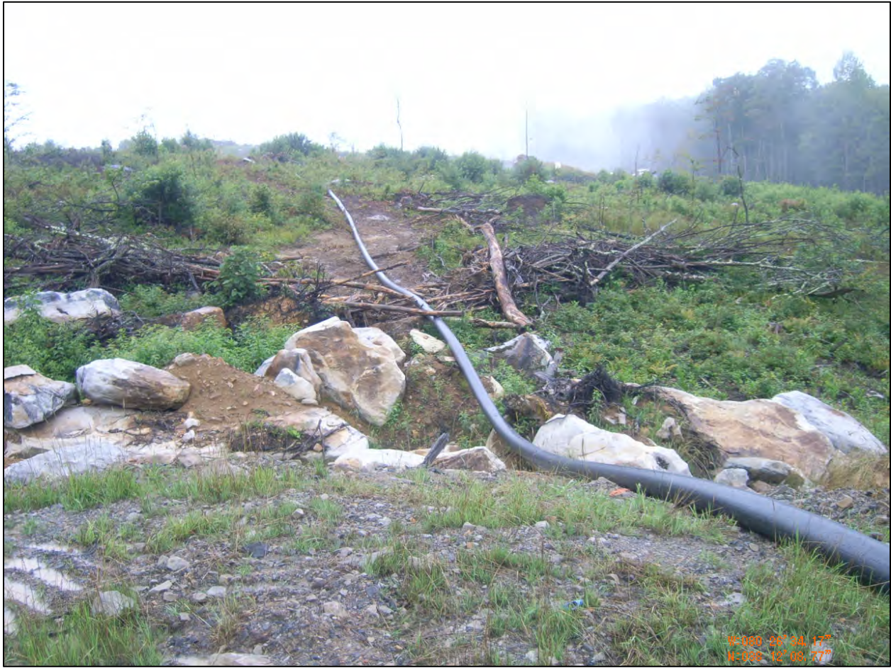
Figure 19: Unsupported Pipe at Plum Creek
