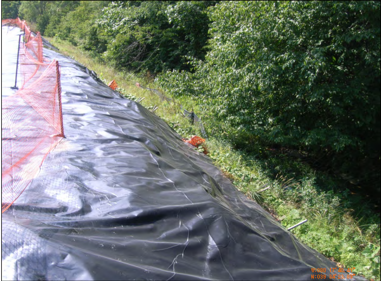
Figure 5: Bulges on Downstream Face
