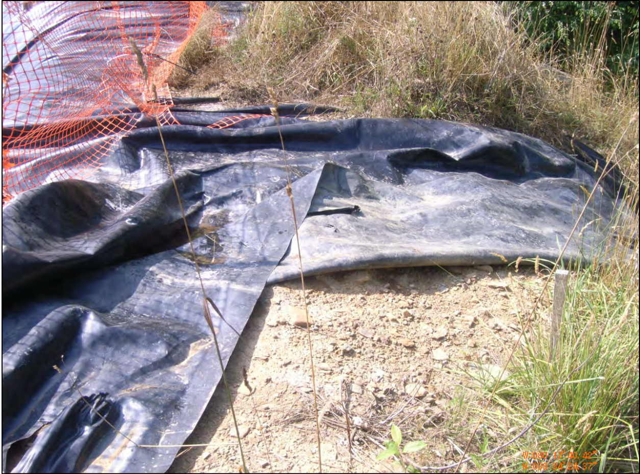
Figure 9: Anchor Trench Exposed
