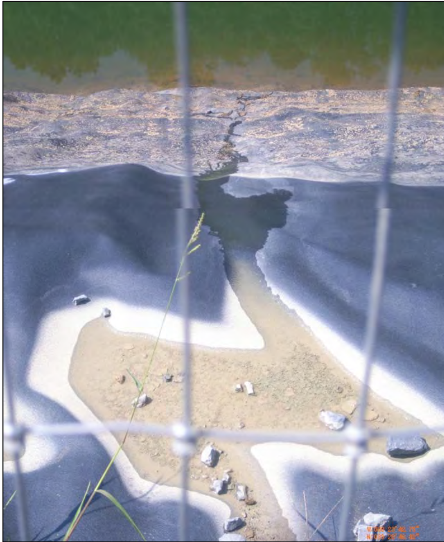
Figure 17: Debris on Liner at Flanigan
