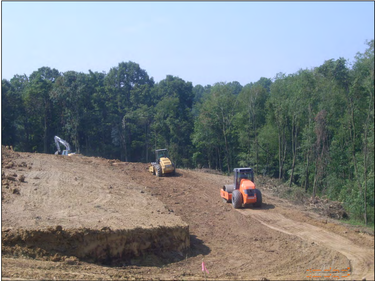
Figure 20: Improper Compaction Practices
