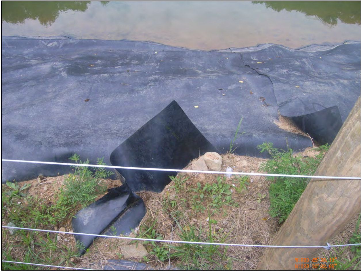
Figure 18: Improper Anchor Trench Embedment at Ball 1H
