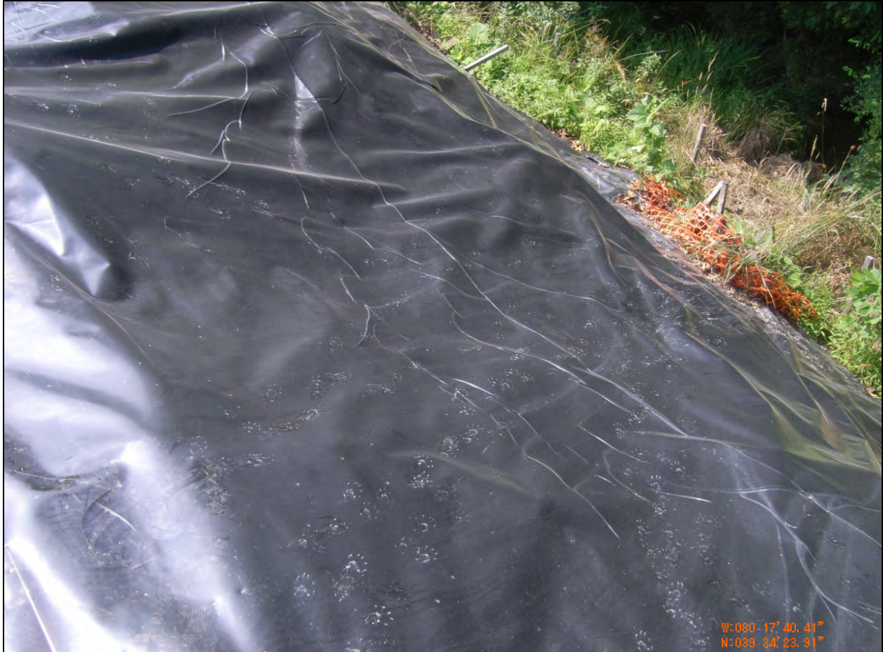
Figure 11: Downstream Slope Movement into Ditch
