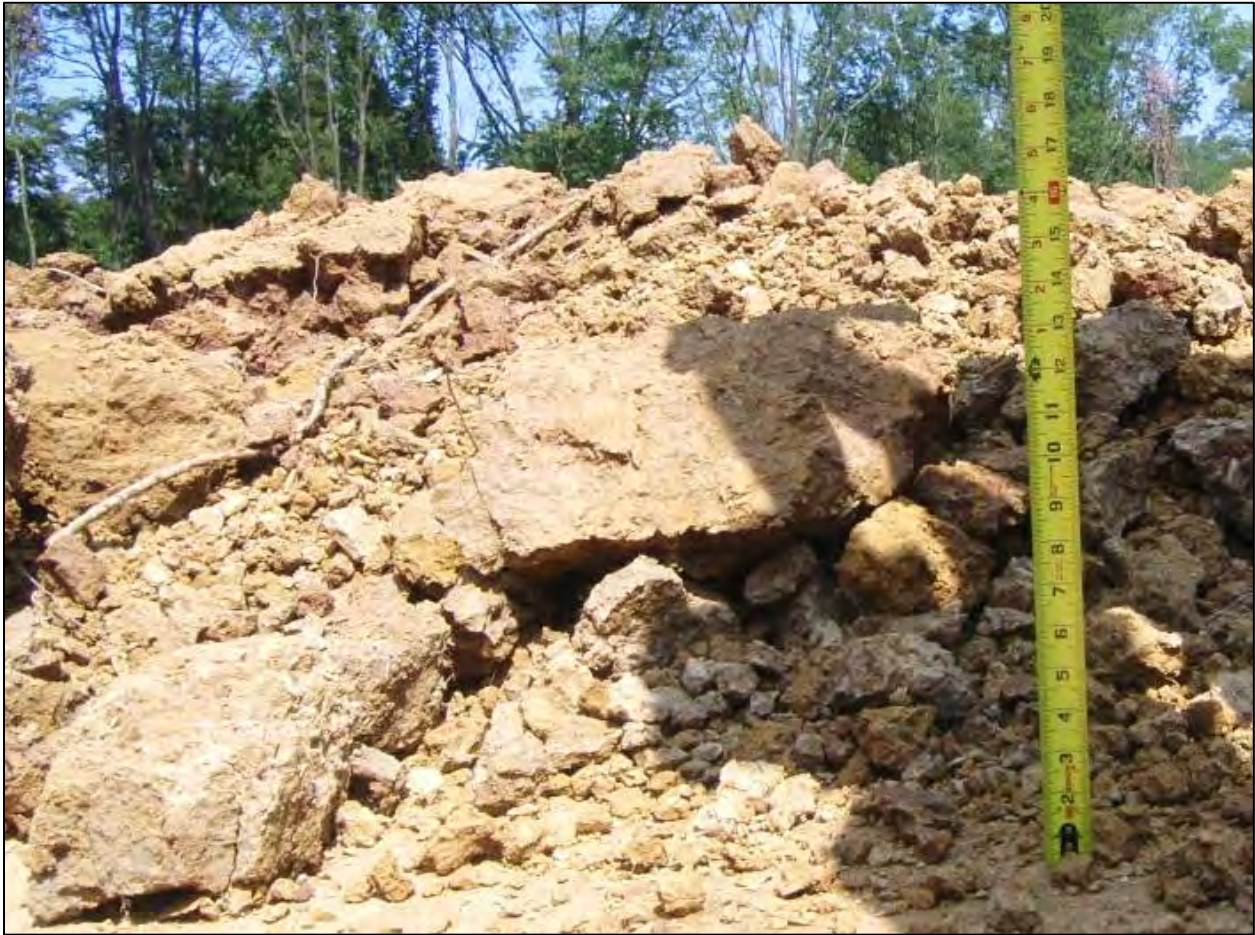
Figure 22: Excessive Lift Thickness
