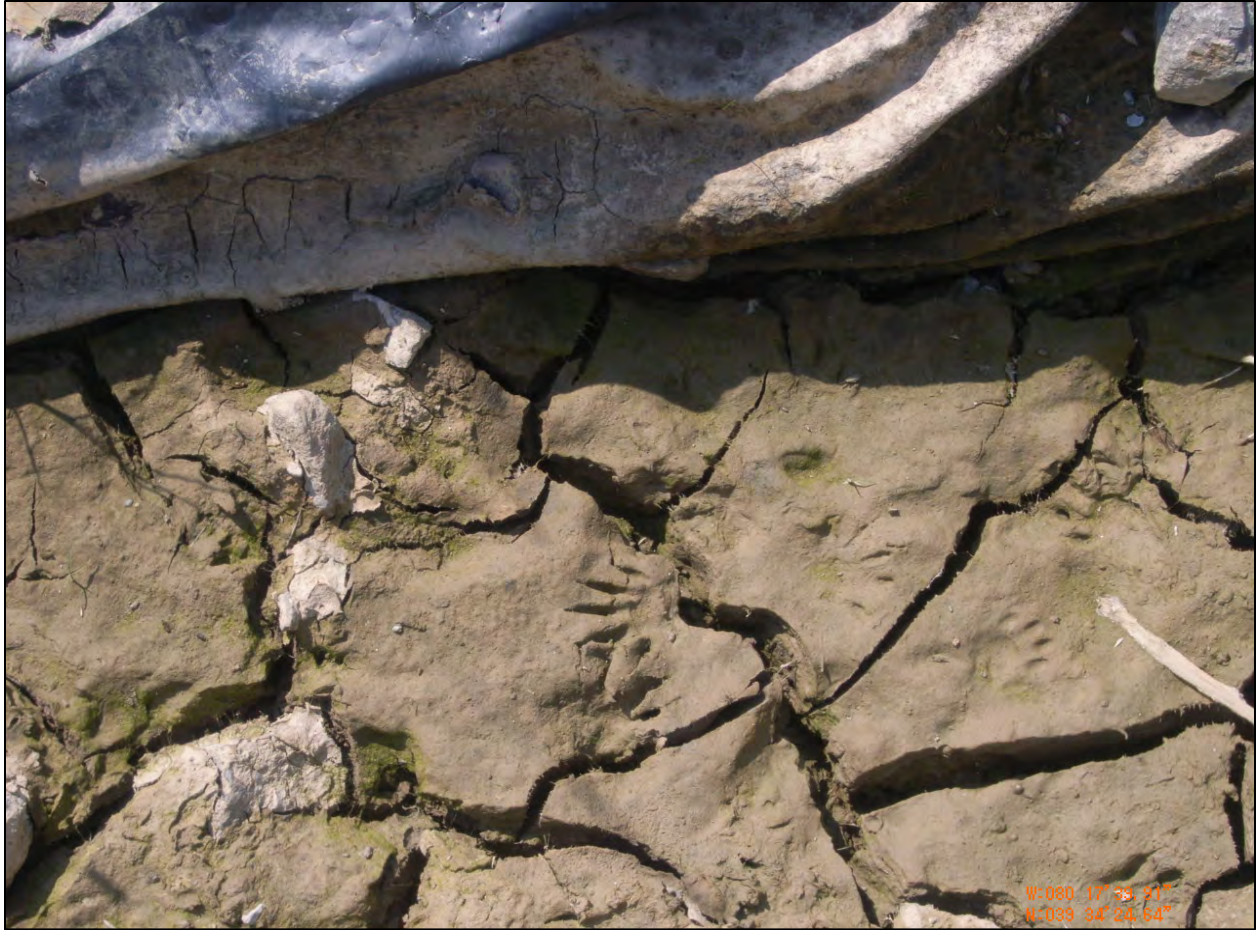
Figure 4: Settlement Cracks in Anchor Trench
