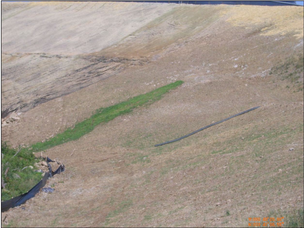
Figure 15: Seepage at Pribble
