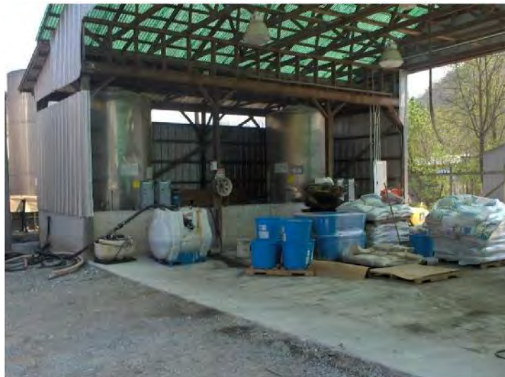
Secondary containment at a bulk pesticide facility
