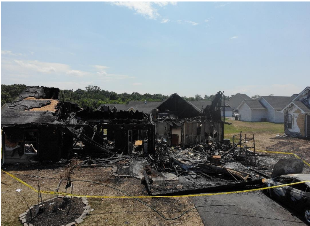
Berkeley County/Photo by ASFM Harms
