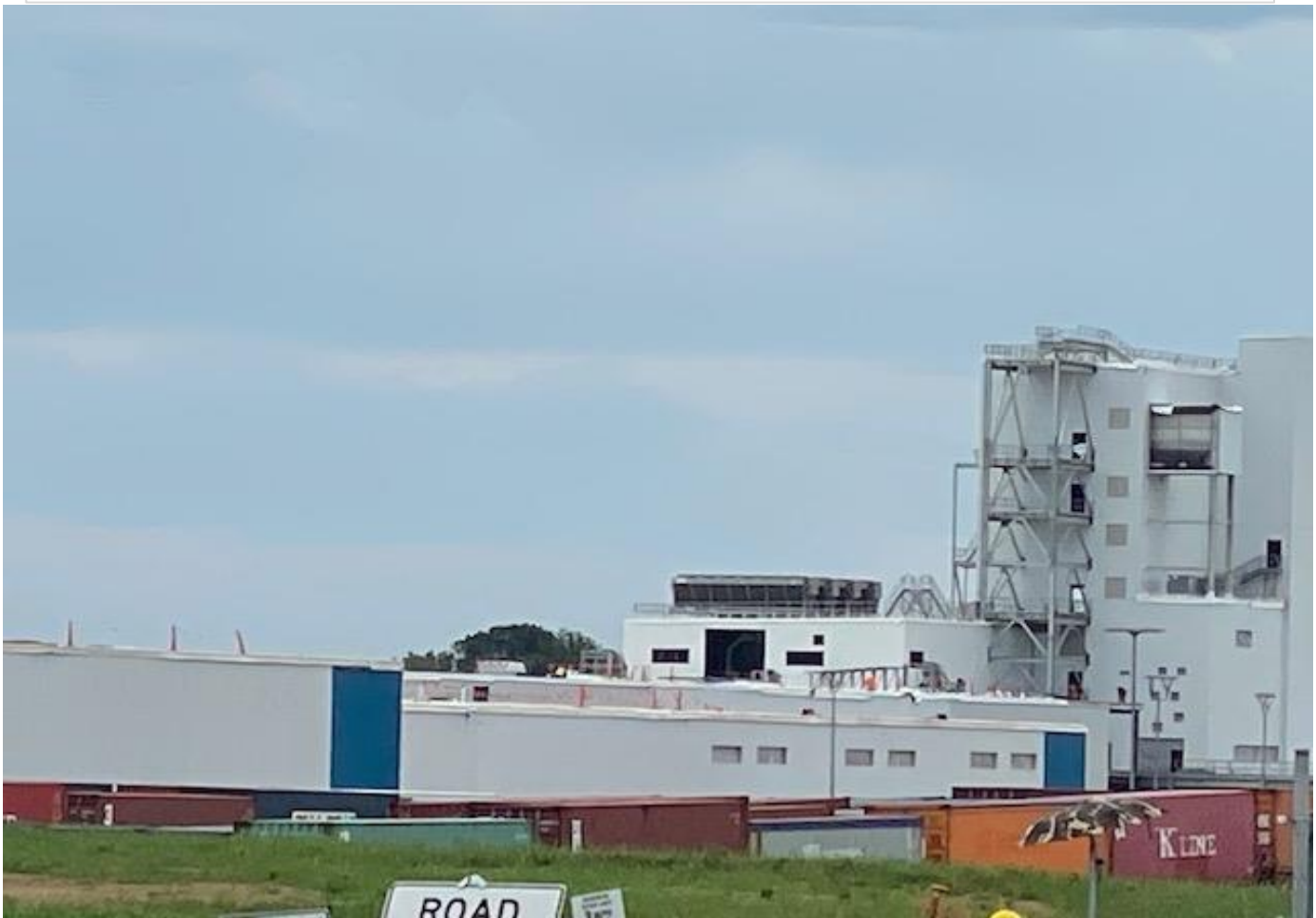
Rockwool Insulation Manufacturing Company - Ranson
