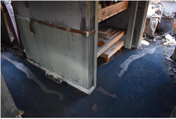
Preston County/Photo by ASFM Sovastion
