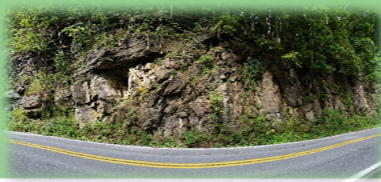
Fault in the Alderson Limestone along Route 39, Pocahontas County
