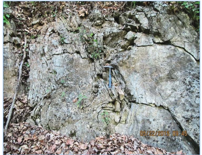
Deformation in the Wills Creek Formation (Photo: RR McDowell)
