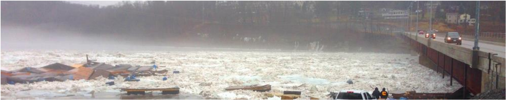
Debris and melting ice damming against the Ices Ferry Bridge on Cheat Lake, March 4, 2015
