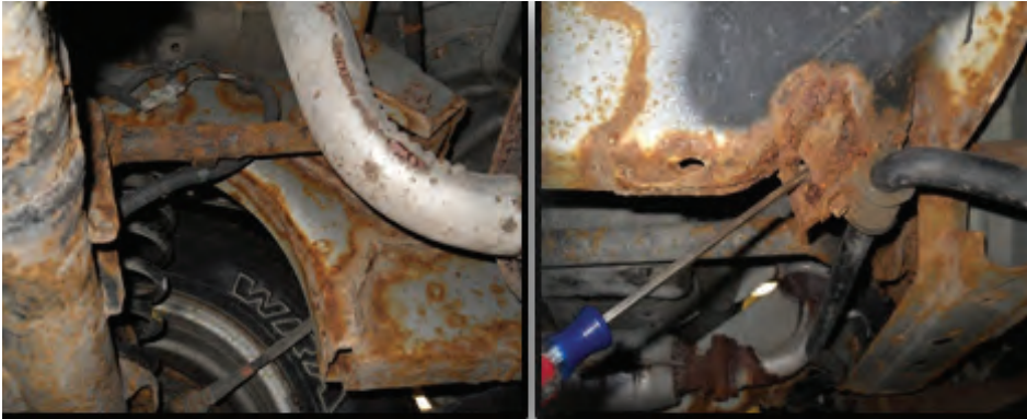
Figure 1 Photographs of Corrosion on Underutilized Vehicles From West Virginia Univesity
