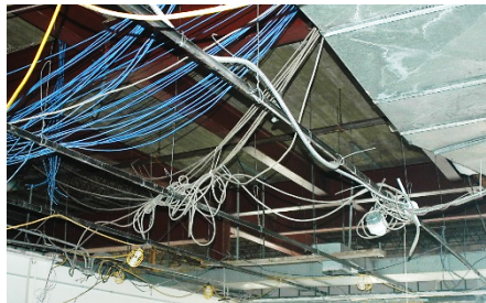
Figure 2 - Floor 6 of Building 4
