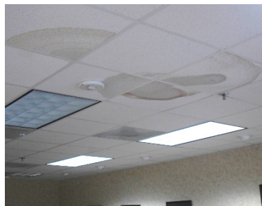
Figure 6 - Areas of leaks on top floor of Building 86
