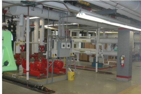
Figure 5 - Energy Saving Project on Floor 11 of Building 5
