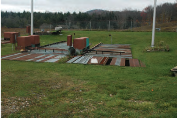
Figure 7. A waste water treatment plant at Canaan Valley Resort State Park. Photo: Performance Evaluation and Research Division.
