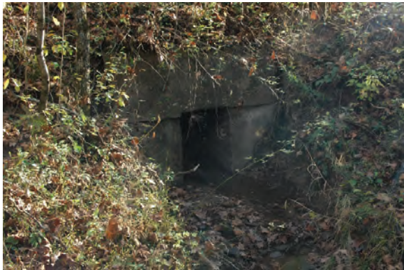
Figure 6. An example of the stone culverts along the North Bend Rail Trail. Photo: Performance Evaluation and Research Division.
