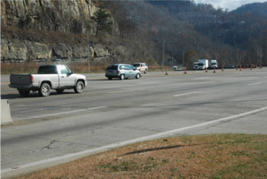
Figure 4 Toll Entrance at Toll Plaza C near Chelyan
