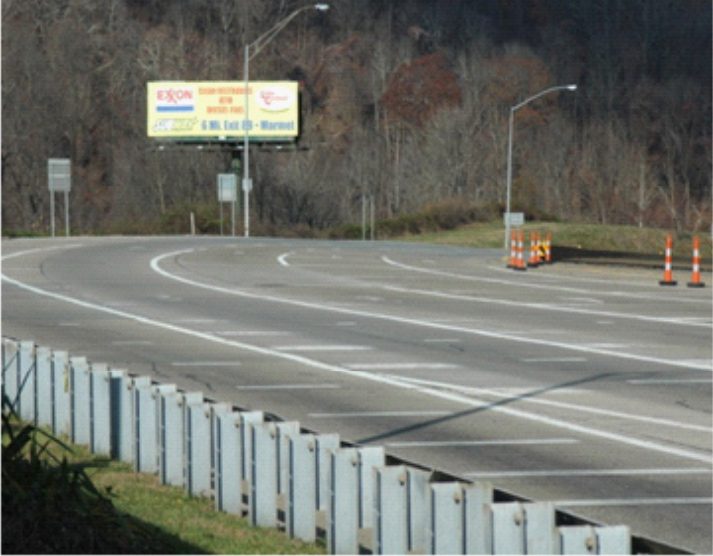
Figure 3 Toll Entrance at Toll Plaza C near Chelyan
