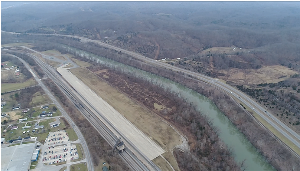
Figure 2 Aerial View of the HIG Facility
